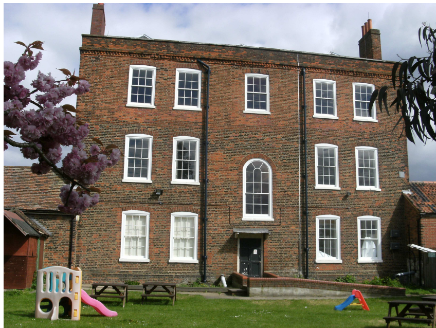
Bretons Manor House Windows
